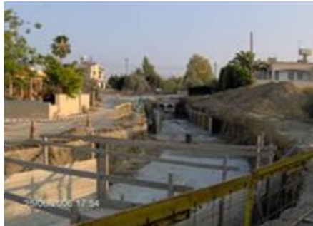
Picture 20 Flood control projects in the Community
