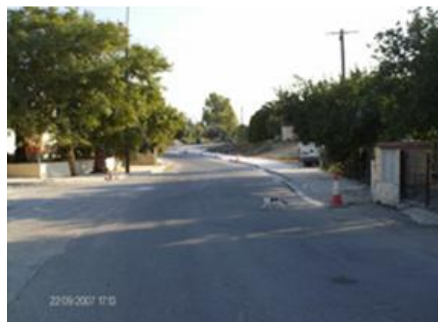
Picture 21 Flood control projects in the Community
