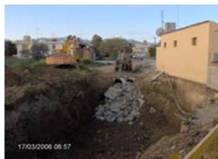
Picture 19 construction stormwater culvert
